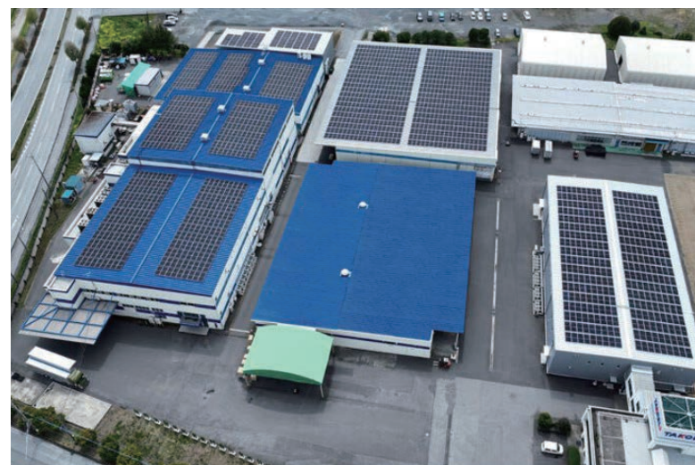
Panoramic view of facility after installation
